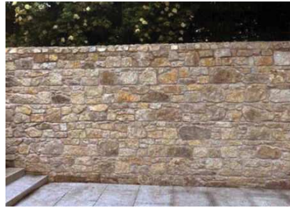
— Stone wall will lower gate to maintain views to the tower. Proposed height: 1.8m
